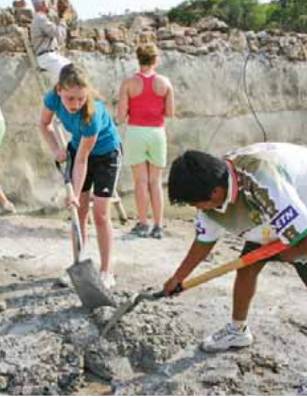
Grace Guyol and Leah Anderson help mix cement for a dam project underway near Galvanes for two decades. The students from the U.S. join Mexicans in working on the dam each year.
